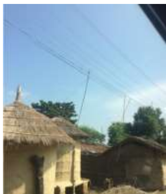
Figure 6: Cable hooking at Paterwa Sugauli – 4
