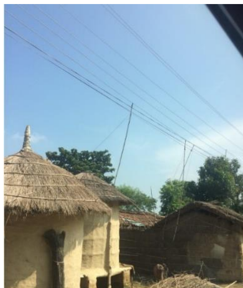
Figure 10: Electrical hooking at Paterwa Sugauli-4 of Parsa DCS (observed during field
